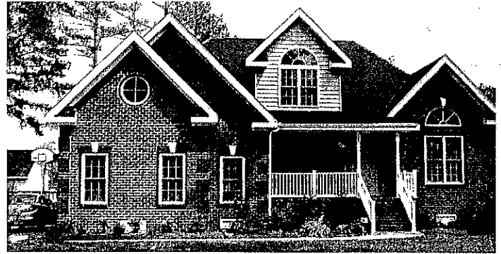
Elevated home on crawl space foundation
