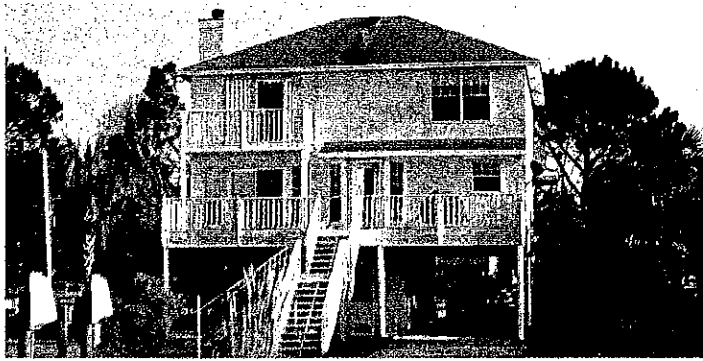
Elevated home on pile foundation
